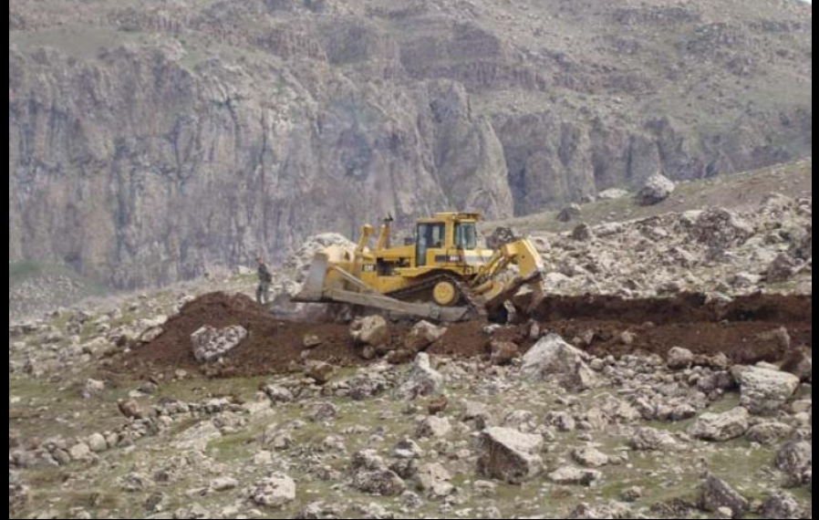
Line clearing for 2D dynamite acquisition
